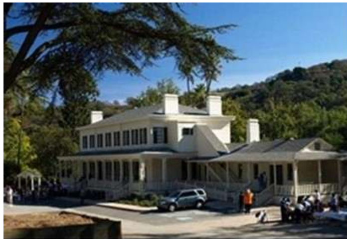
Casa Grande After Restoration, Nov. 11, 2010, Ron Horii Photo
