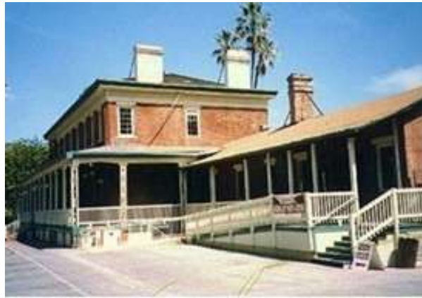
Casa Grande Interpretive Center, Prior to Restoration, circa 1999
